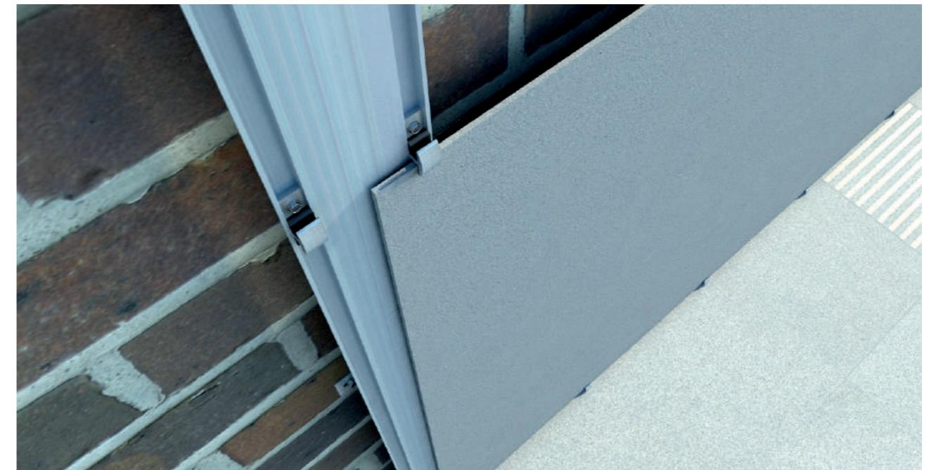
The staples to mechanical fixation are made of extruded aluminum from aluminum-magnesium-silica allow quality 6063 (Al Mg Si 0,5), with T-5 treatment.
