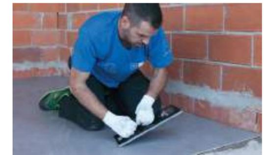
The beating operation is then carried out for the readjustment of the sheet and to form in this way a uniform and well compacted layer of adhesive. For this operation, a manual or mechanical rubber trowel is used.
