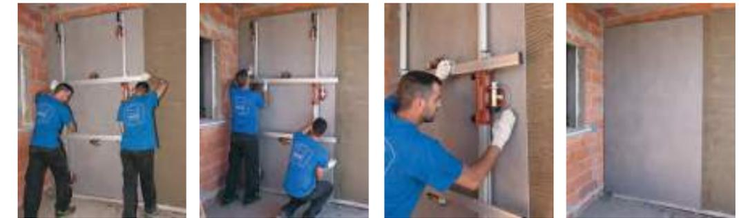
ADJUSTING THE PARTS/ AJUSTEMENT DES PIÈCES
