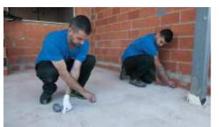
To proceed with the gluing of the ARKLAM sheet, the double gluing method is used:
