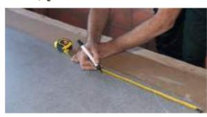
Prior to the completion of the cut and the ARKLAM piece, proceed to the marking of the cut line, place the guide and fix
