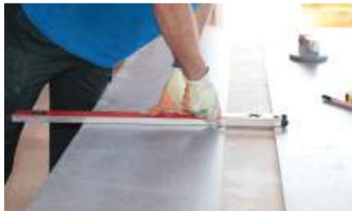
For the cutting of small pieces or reduced lengths, the manual diamond pencil can be used.
