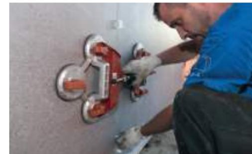
Combined with this system, the distance between plates will be adjusted by using manual suction cup systems.
