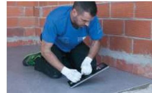
The beating operation is then carried out for the readjustment of the sheet and to form in this way a uniform and well compacted layer of adhesive. For this operation, a manual or mechanical rubber trowel is used.
