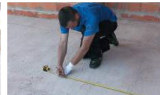
In addition to the general delivery conditions of the laying surface, a flatness of the laying surface of 1.5 mm measured with a 2-m ruler must be requested for the laying of ARKLAM.
