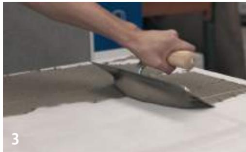
Apply adhesive on the back of the ARKLAM sheet using a flat trowel or if necessary by means of a 3 mm notched trowel, in a horizontal pattern.
