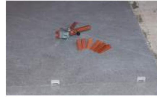
To proceed to the correct levelling between plates, a reference is always taken from the levels of the previous plate. The system of wedges in the union between the newly installed plate with the previous one is used.
