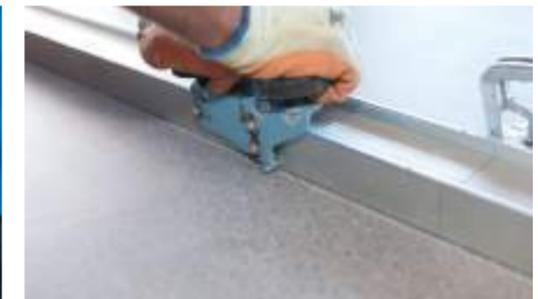
For the execution of a dry cut of the ARKLAM piece, cutting guides with suction cups are used. The guide will be set and its position fixed.
