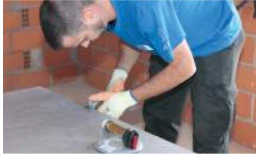
Once the scratching has been done, by means of a pair of pliers, we proceed to the partition of the pieces on both sides of the cut, applying pressure at a suitable point until it breaks. Keep in mind that there must be one or two people holding the piece so that it does not fall.
