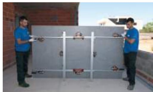
Prior to positioning the suction cups on the ARKLAM sheet, wipe the surface and the grip of the suction cups with a damp cloth so as to ensure better adhesion.
