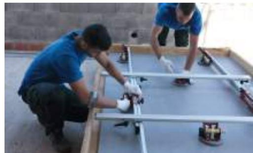
For the transport and manual handling of ARKLAM sheets, rigid frames should be used, and it is advisable to use whenever possible an easel with displacement wheels for handling on the same level. Equipped with powerful vacuum suction cups. This manual always refers to the handling of entire ARKLAM parts. For this task, a minimum of 2 workers, using protective and non-slip gloves for glass and safety footwear, is advisable. Keep your spinal column straight when working.
