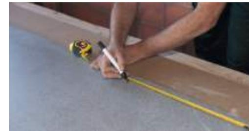
Prior to the completion of the cut and the ARKLAM piece, proceed to the marking of the cut line, place the guide and fix its position.
