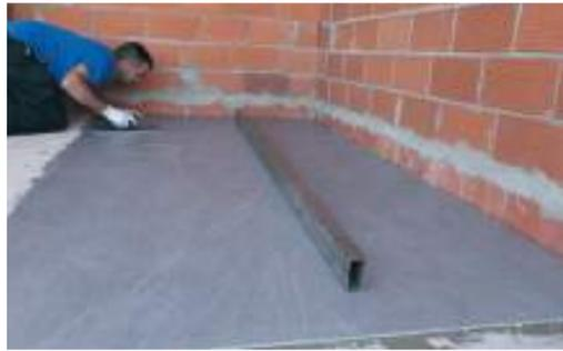
When positioning on a surface, check its horizontal level.
